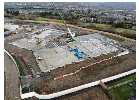
Current progress on site
