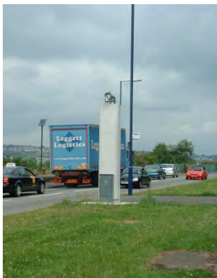
Figure 2.1.5 - St Thomas DOAS Transmitter
