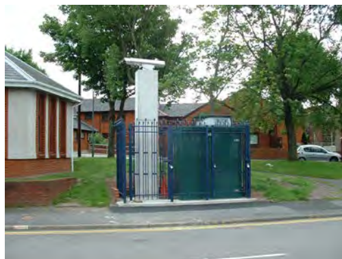
Figure 2.1.6 - St Thomas DOAS Receiver Station
