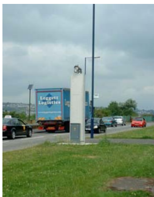
Photo 1 - St Thomas DOAS Transmitter
