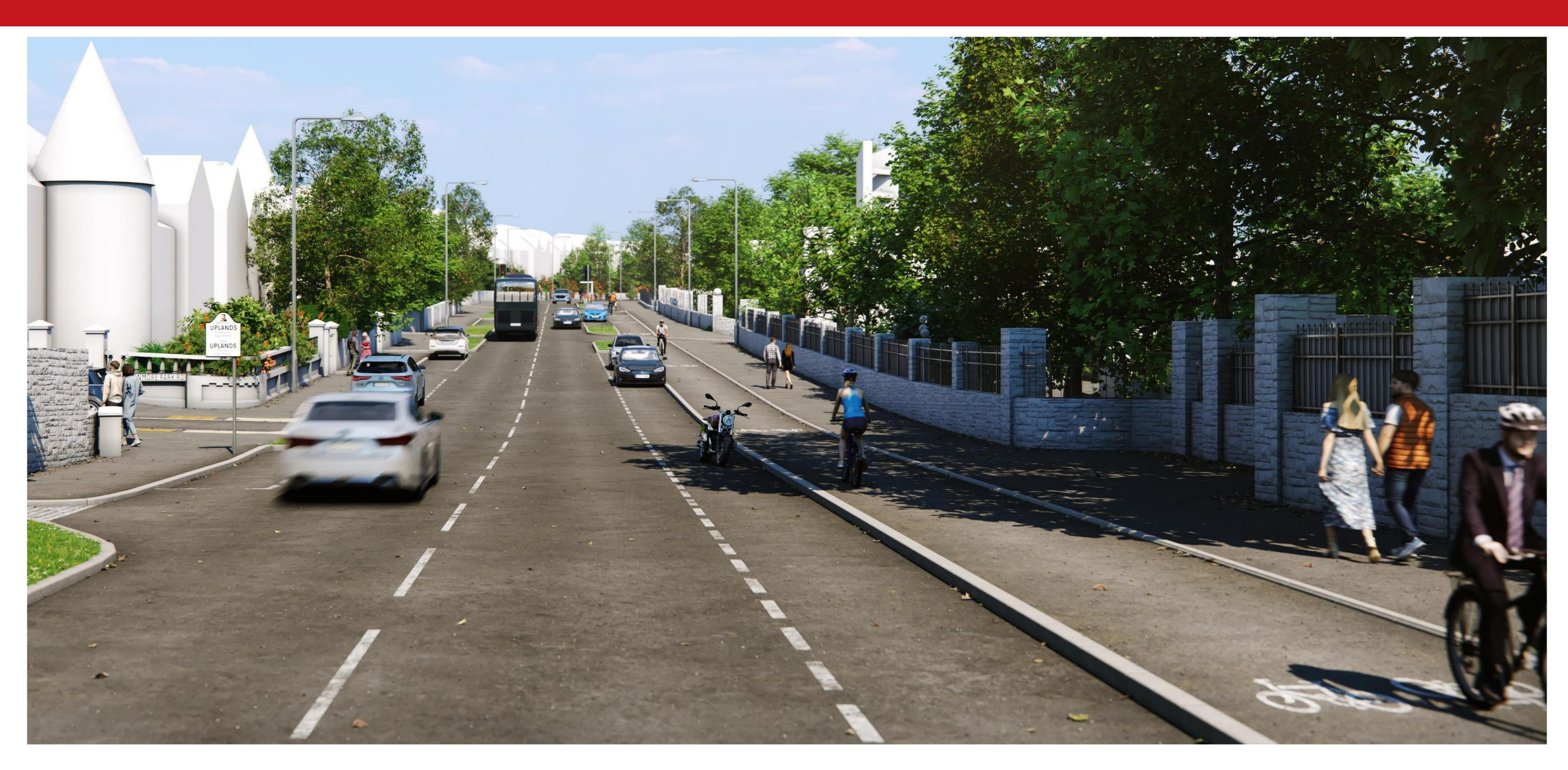
The illustration shows what Sketty Road could look like around the junction of Glanmor Park Road, looking towards Uplands. It shows the proposed two-way cycle track on the south side of the road, alongside an area set aside for parking and the existing central hatched area removed.
